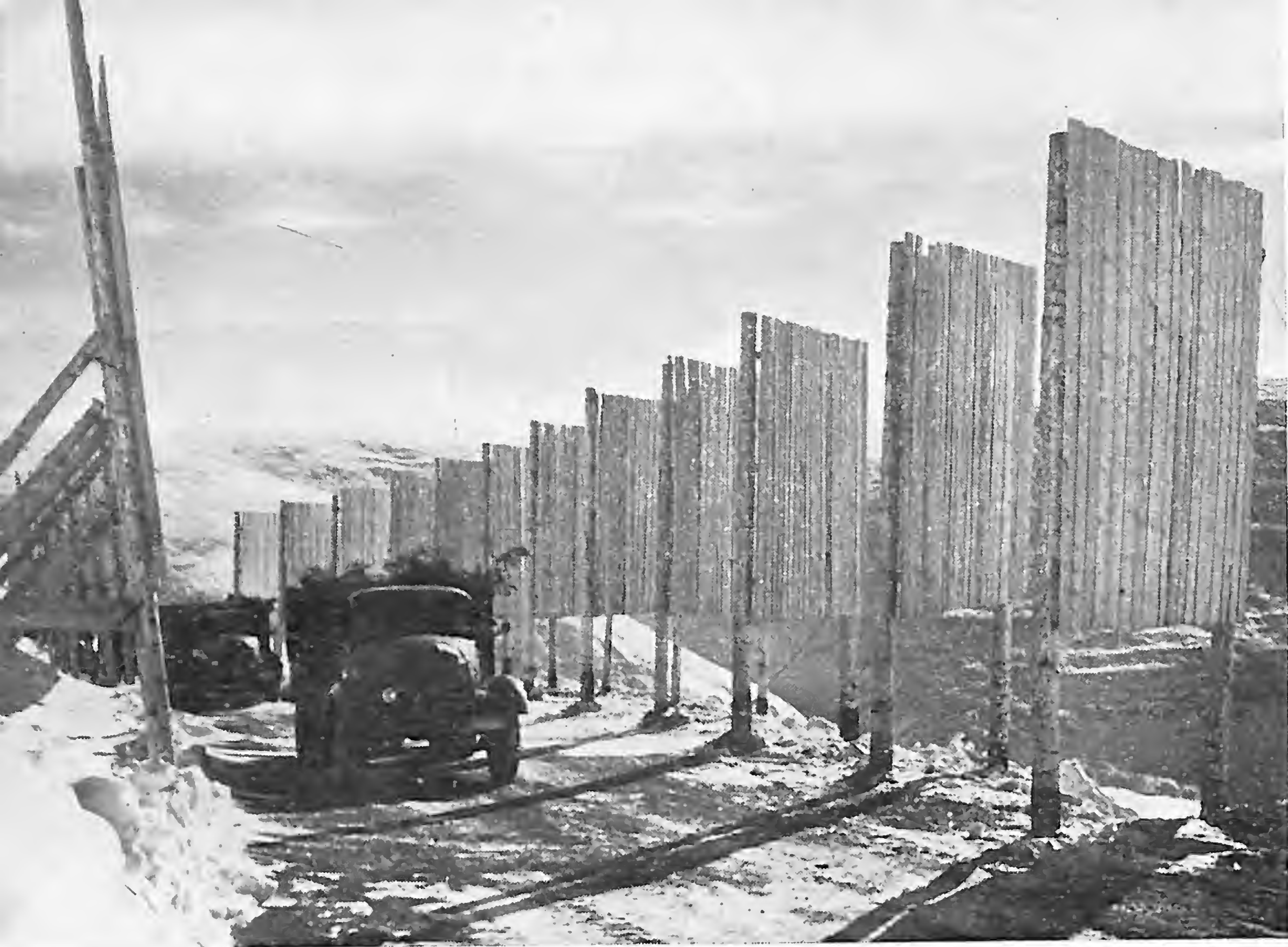
Wind-deflection panels along the highway.
